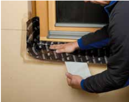
Can be used to create sub-sill flashing.
