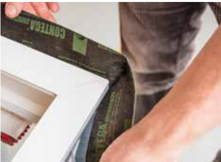
Create loop of slack at corner (length: 1.5 x width of gap).
