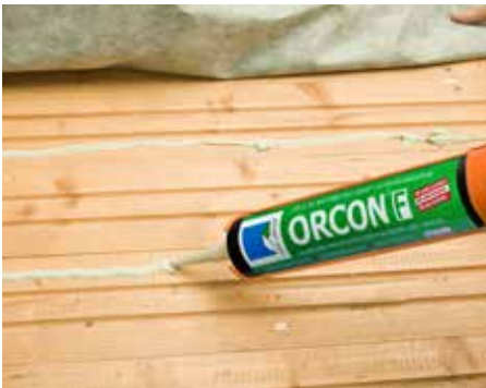
... for vapour checks underneath external roof insulation,
