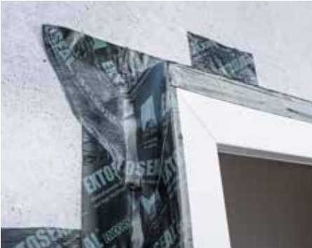
Joints between windows and masonry or concrete structures.
