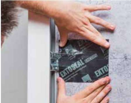
Waterproof taping of angle brackets.
