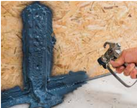
Airtight spraying over angle brackets,
