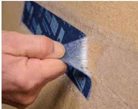
The primer strengthens unstable subsurfaces.
