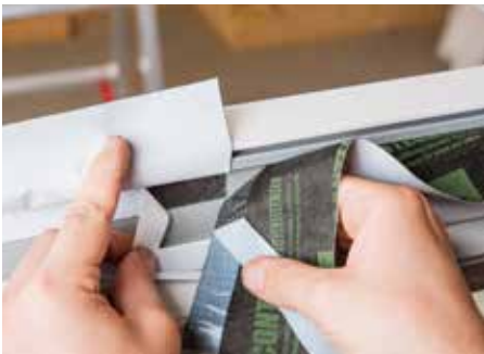
Stick tape ends to one another, length: 5 cm.
