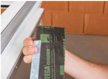
Remove the release film strip.
