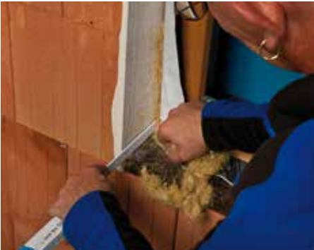
Install the window and insulate the joint
