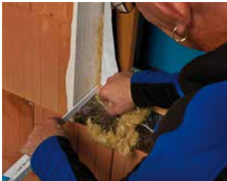
Install the window and insulate the joint
