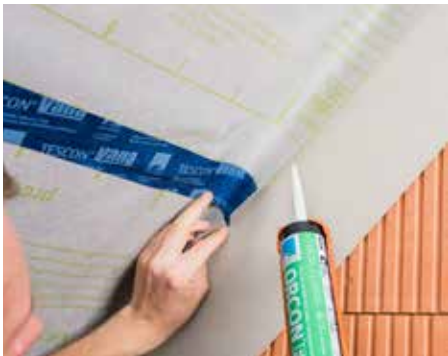
Adhesive sealant for interior airtightness membranes,
