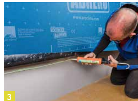
3 Sealing to rough subsurfaces using ORCON F
