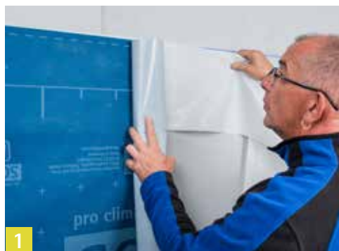
1 The membranes are generally installed horizontally
