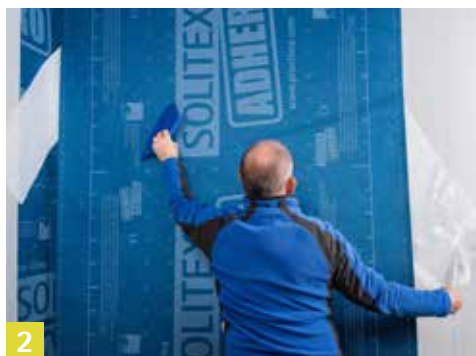
2 Possible alternative: vertical installation
