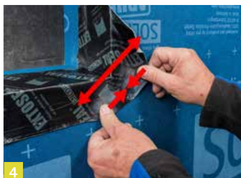
4 Form the sub-sill flashing using EXTONSEAL ENCORS
