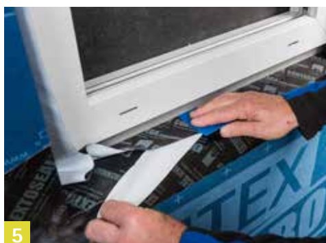
5 Seal the window joints on the inside and outside using CONTEGA
