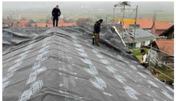
Pre-fabricated sheet of SOLITEX MENTO 5000 connect rolled out on the roof
