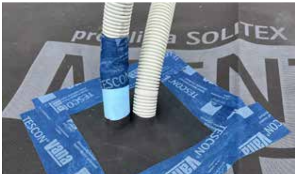
Sealing of penetrations around conduits with the ROFLEX grommet for multiple conduits ...
