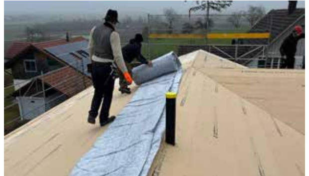
Rolling out of the pre-fabricated cut and bonded underlay membrane
